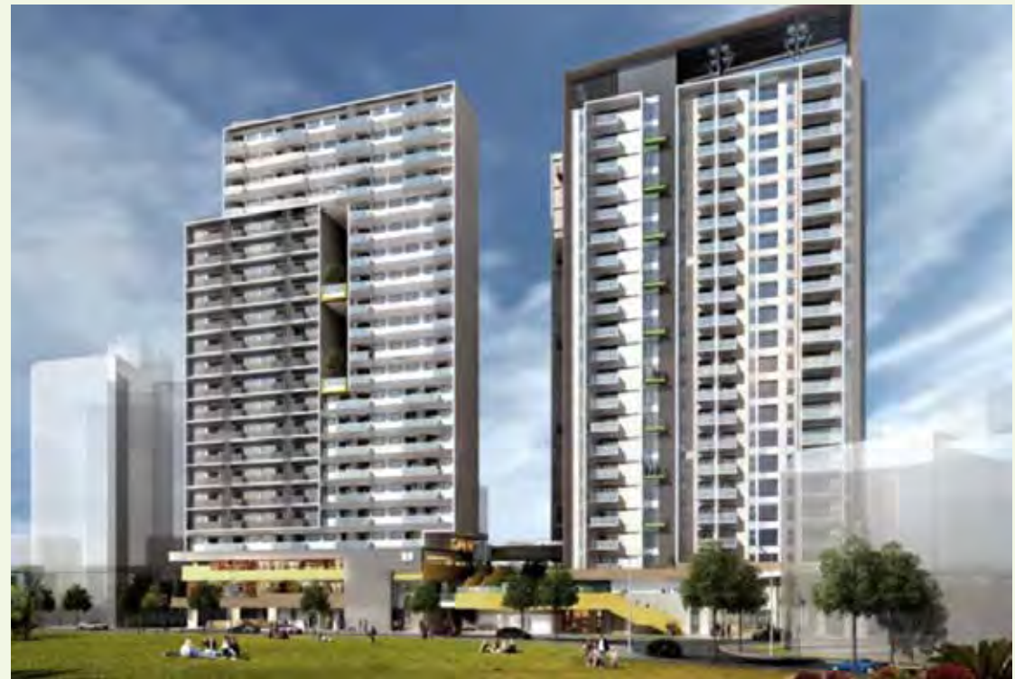
Using Goldsun's concrete in the structure, Jinzhou St.'s social housing is a silver green-rated building.
