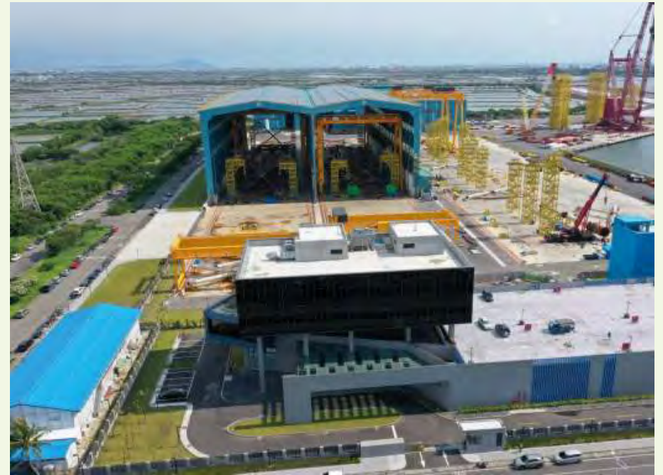
Underwater Infrastructure Plant of the CSC Wind Power Facility at Xingda Port
